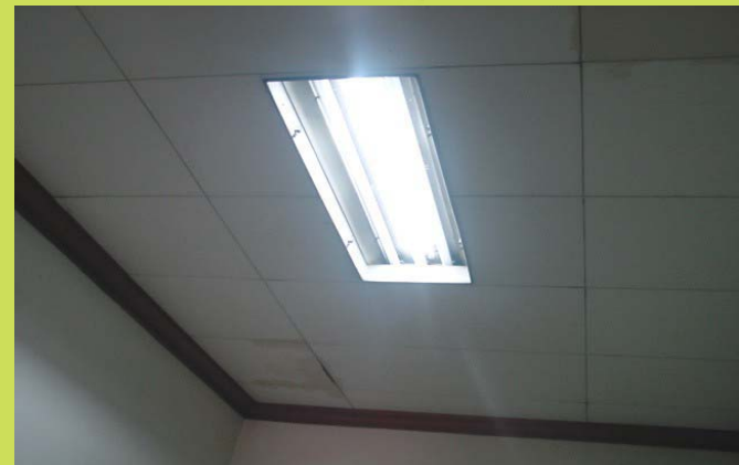
CEILING WITH JOINT
